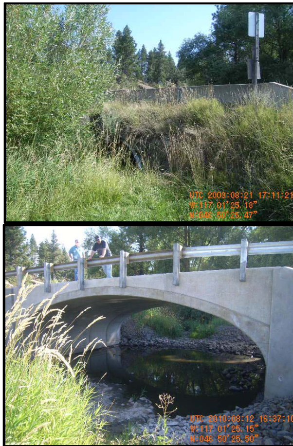
North Viola Bridge – Before and After Flood Mitigation Project
